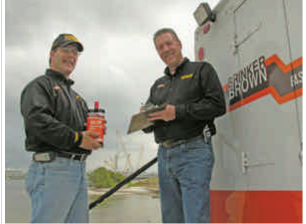
The company's 20/20 epoxy is the product that opened the door to the major bridge project in the background for jobsite specialist DJ Uman, left, and sales manager Tom Barklow.
